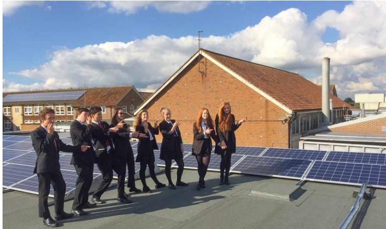
Students at Ringmer College inspect their new solar panels, installed by OVESCO
